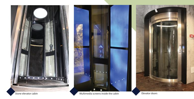
six photo and video displays are mounted in the cabin, making it possible to modify the media show whenever desired. The panoramic cabin is circular with glass walls and doors, capacitive control and a transport capacity of eight passengers (600 kg).
